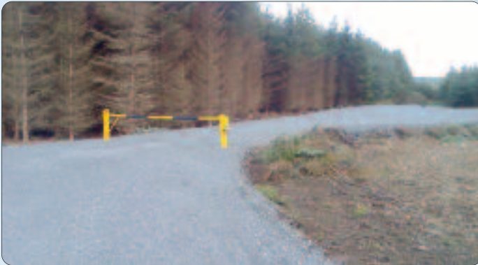
Completed harvest road for 5FIP site at Brosna, Co. Kerry
